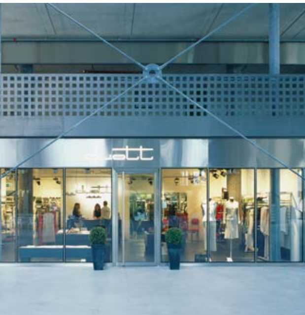
Fire resistant door and fire resistant glazing T30/F30 – Puls 5, Zurich, Switzerland
