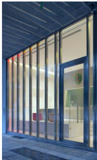
Burglar resistant door and glazing in stainless steel – Belgian Embassy, Athens, Greece
