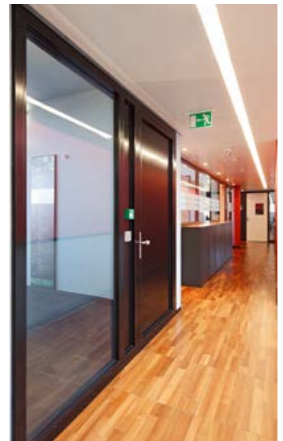
Burglar resistant thermally insulated glazing – KBA NotaSys, Lausanne, Switzerland
